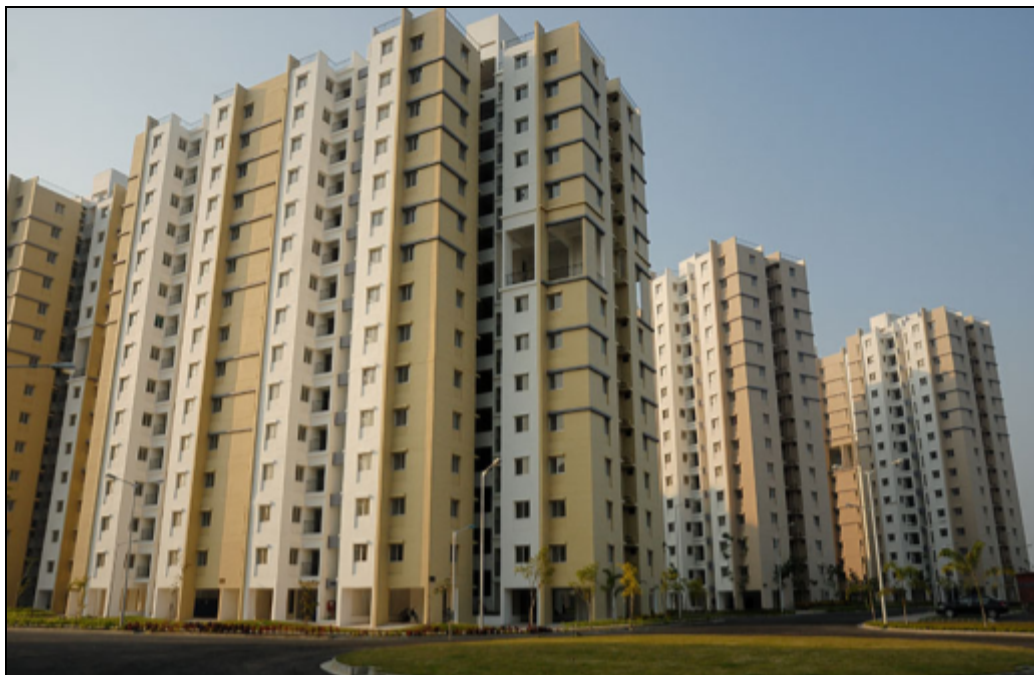
Figure 17: Example of a housing complex. Source: http://www.shukhobrishti.com/gallery
